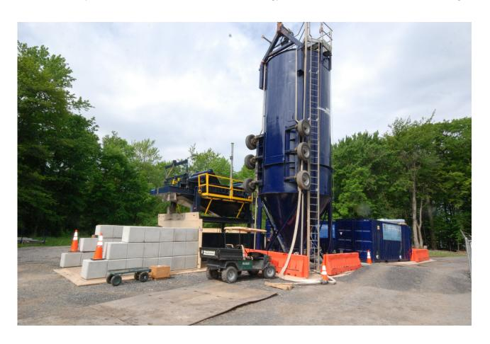
Process Piping & Electrical Connections On The Pad Are Provided and Installed by MPS Technicians Process Pad Lay-down Area 96' L x 28'W 42' H
